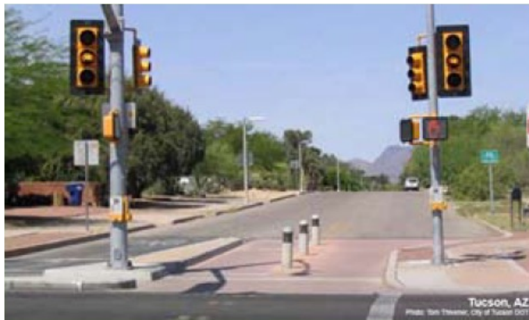
■ FIGURE 3-9 Tucson, Arizona, first bicycle signal
