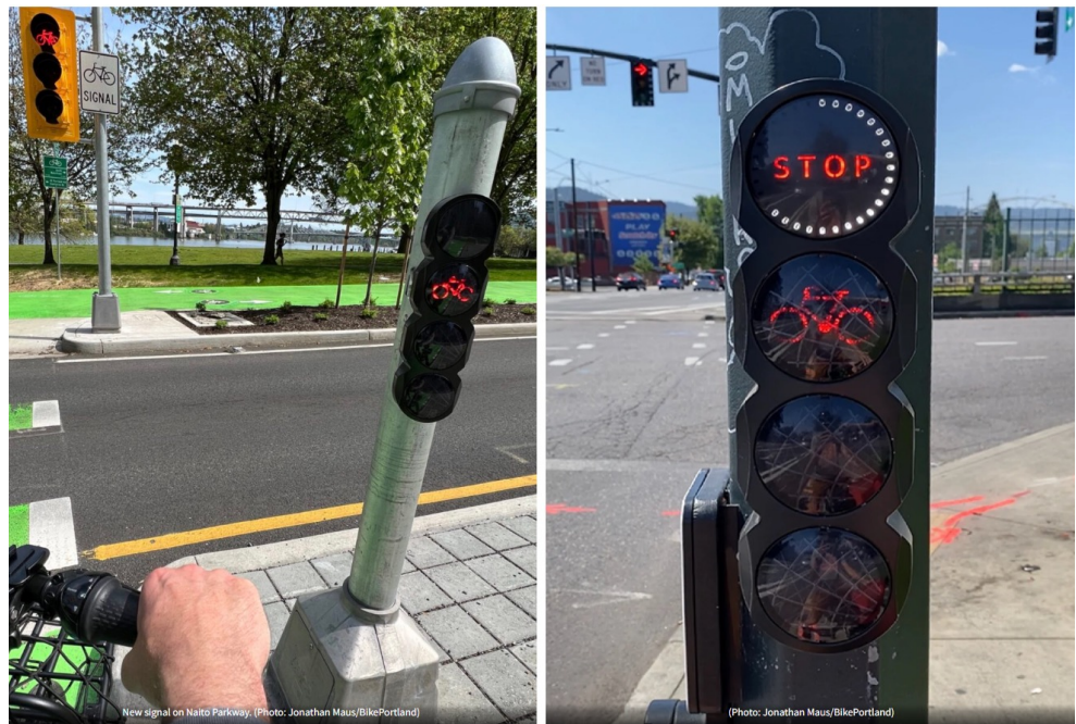
■ FIGURE 3-4 New type of bicycle signal imported from the Netherlands to Portland
