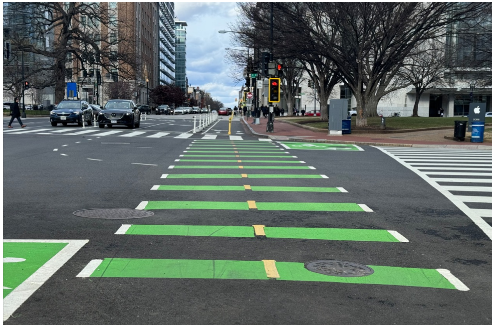
■ FIGURE 3-7 Example of bicycle signals and infrastructure in Washington, DC
