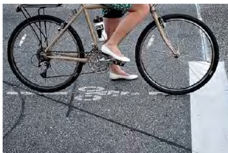
■ FIGURE 2-6 Passive bicycle detection pavement markings
